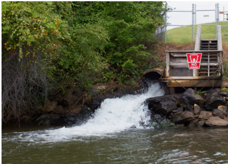
An outfall dumps contaminated water from a Duke Energy coal ash pond into Lake Wylie in Charlotte, North Carolina; this practice is permitted under state law.
